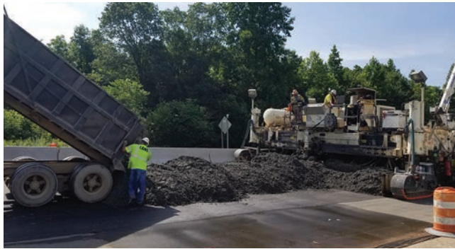
Figure 5.15. Uniform deposition of concrete in front of the paver
