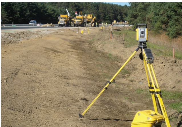
Figure 5.5. Stringless paving system guidance using total stations
