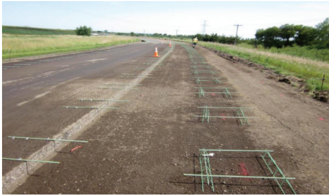
Figure 5.18. Preplaced tie bars supported and fastened to the grade
