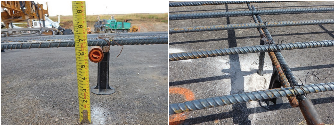
Figure 5.8. Verification of positioning of reinforcing bars for CRCP and support conditions (left) and staking of reinforcing bars to subgrade (right)
