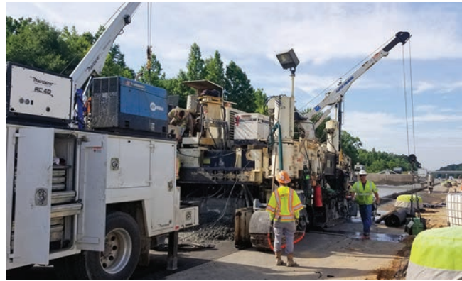
Figure 5.16. Maintenance truck (at left) with tools and equipment available to address issues with the paver during paving
