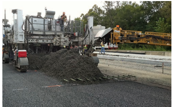
Figure 5.7. Preplaced dowel baskets fastened to asphalt base, with markings located on base to guide sawcutting
