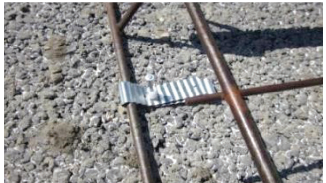
Figure 5.6. Dowel basket anchored to subgrade (top) and existing asphalt (bottom)
