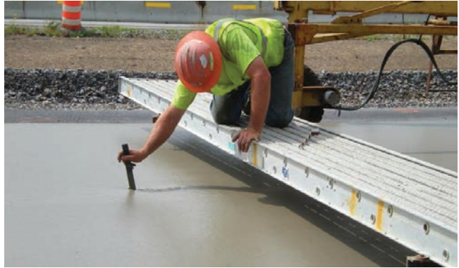
Figure 5.19. Verification of dowel bar location by probing behind the paver
