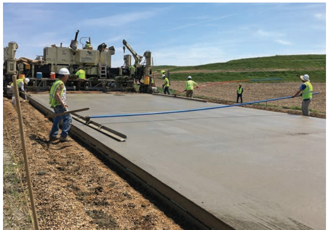
Figure 5.20. Hand finishing
